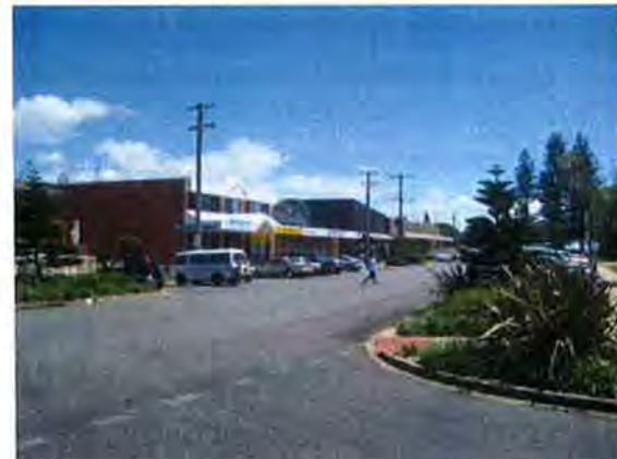
Picture 4 – Queen Street (northerly aspect)
